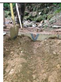
Weir during construction
