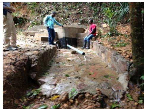
Completed spring box
