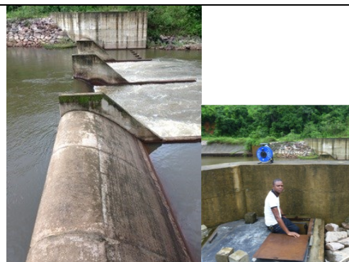
Ogee crest weir and stilling well
