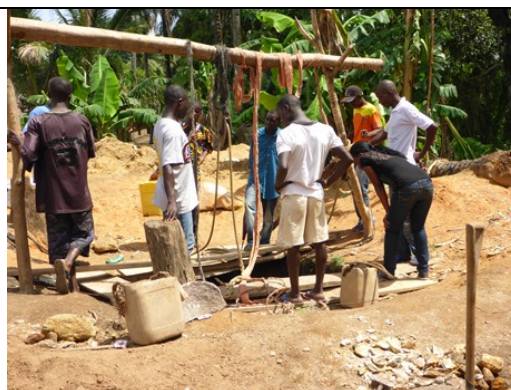
New well under construction
